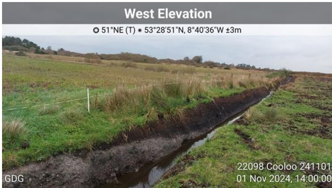
Figure 2-3: Peat and superficial deposit transition exposed in trench - east of Substation location
